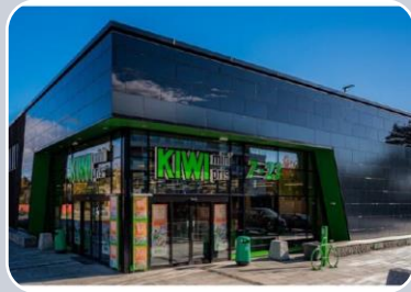
Building- integrated PV (BIPV)
