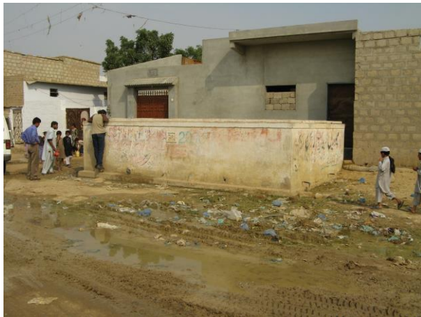
Orangi Awami Tank
